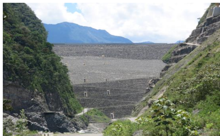
The dam across the Río Huallaga, Chaglla hydroelectric project
