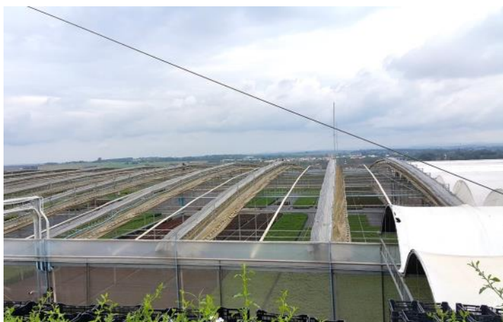
Opening retractable greenhouse roof by sections
